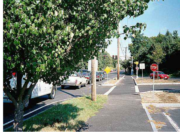
Trees interfere with cyclists' line of sight on this path
