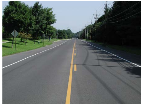
Bicycle compatible shoulders on South Mill Road
