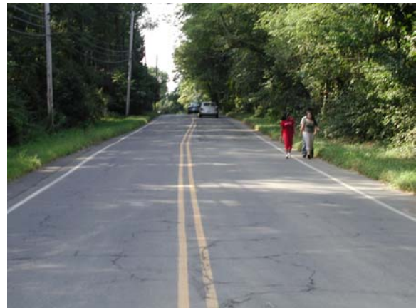
Lack of sidewalks on Millstone Road
