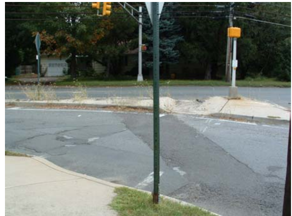
Faded and worn crosswalk
